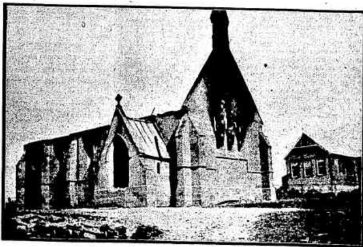
The walls and porch of building as they appeared after the fire which destroyed the whole of the contents yesterday morning. The new Stations of the Cross, recently provided at a cost of £200, and the valuable stained-glass windows, which were destroyed, renders the loss the more severe. The building on the right, which escaped the flames, is used as a Sunday school.
